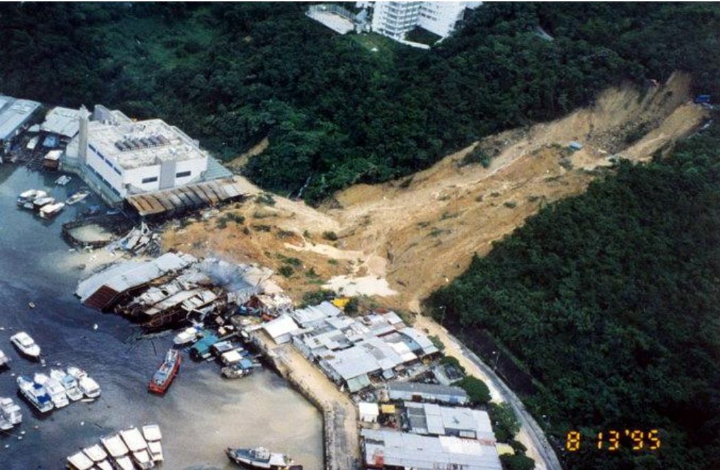
Deslizamiento de Shum Wan Road, HK
